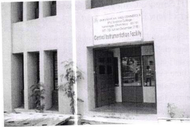
External View of CIF Centre
